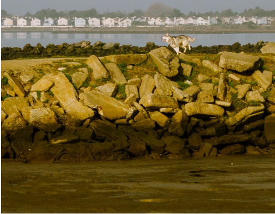
Figure 7 - An example of 'fortification' at Point Isabel, Contra Costa County (photo by Shira Bezalel, 2015).
