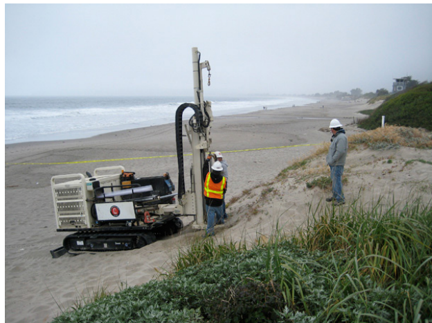
Figure 6. Geophysical contractors use a drill rig to install monitoring wells at Stinson Beach, Calif. Image from: https://news.stanford.edu/news/2010/may/septic-wastewater-sea-052010.html
