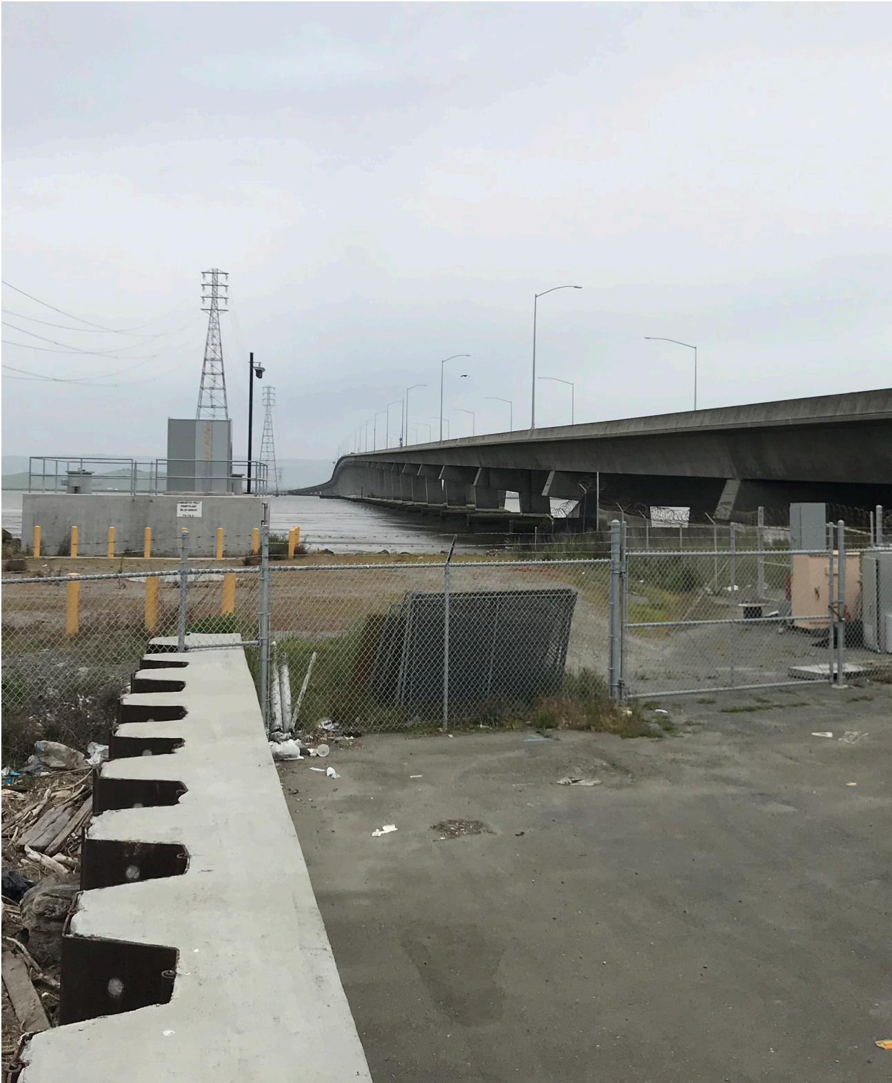
Local access roads near the SR-84 Dumbarton Bridge touchdown. A temporary barrier exists to provide short-term flood protection. Photo by BCDL.
