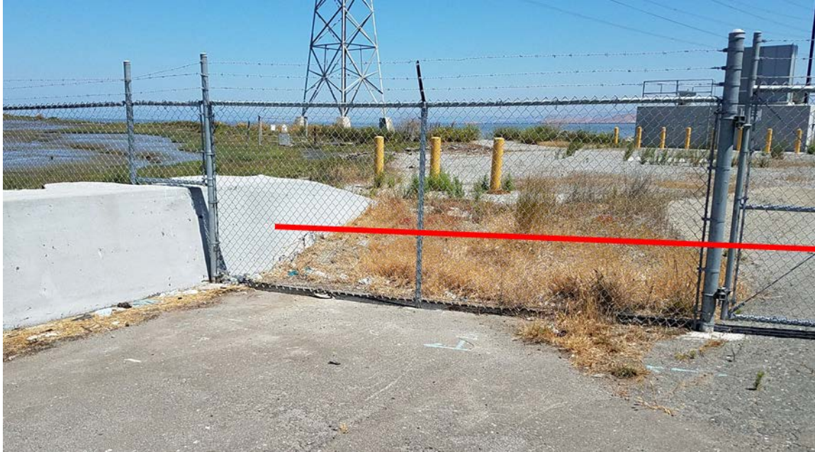
Figure 13. Location of gap in flood protection system at east pump station.
