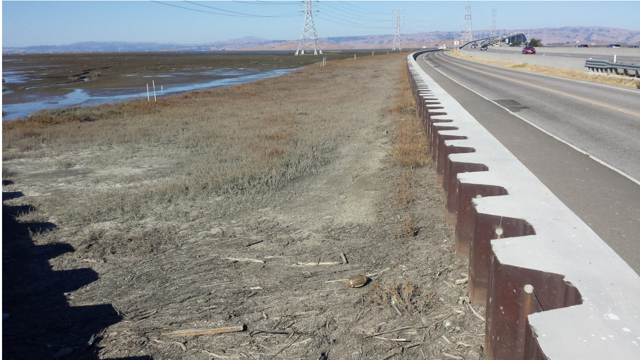
Figure 2. Sheet pile wall and concrete barrier on edge of north access road. Image is looking east, towards Dumbarton Bridge and the Bay.
