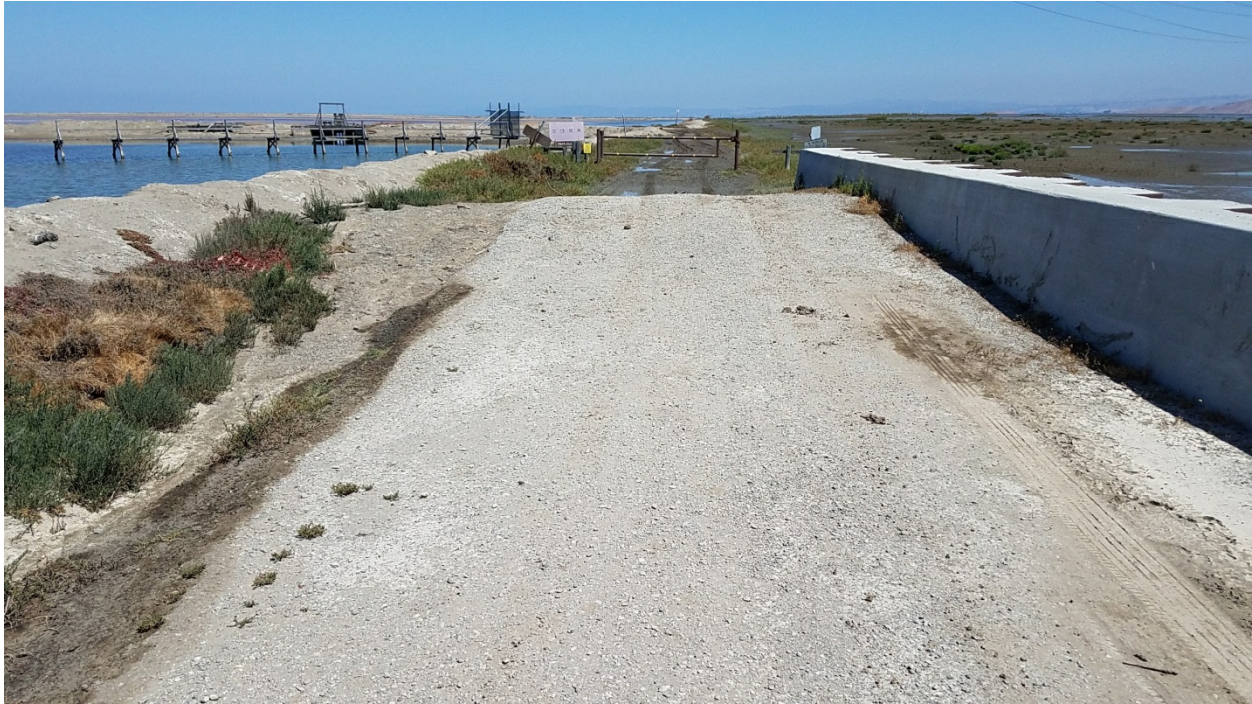
Figure 4. Cross berm along crest of N-S levee and concrete barrier. Photo is looking north.
