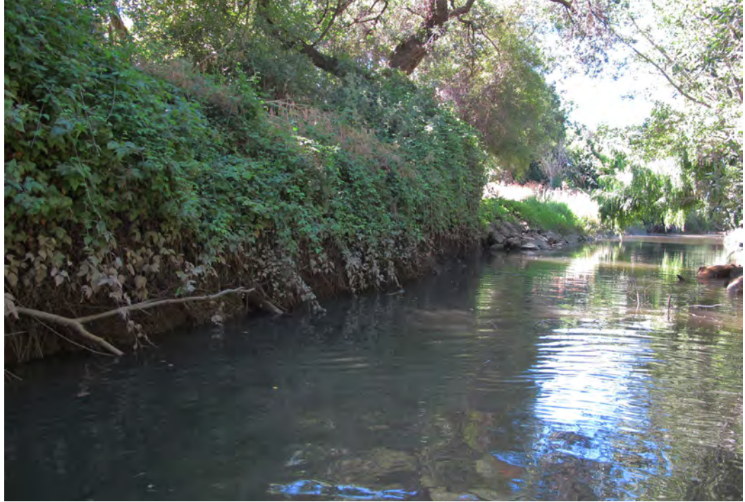
Figure 3.20. Coyote Creek tidally desiccated vegetation line. This photo shows desiccated vegetation indicating that this reach is still under tidal influence.
