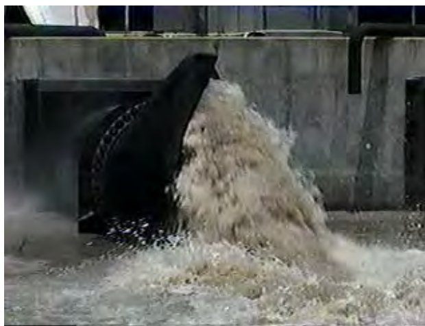
Figure 5. Duckbill check valve discharging water. Photo credit: Tideflex Technologies.
