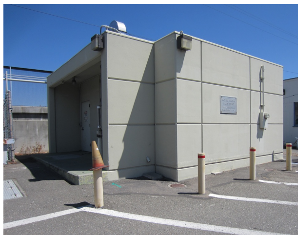
Figure 4. EBMUD’s pump station G.
