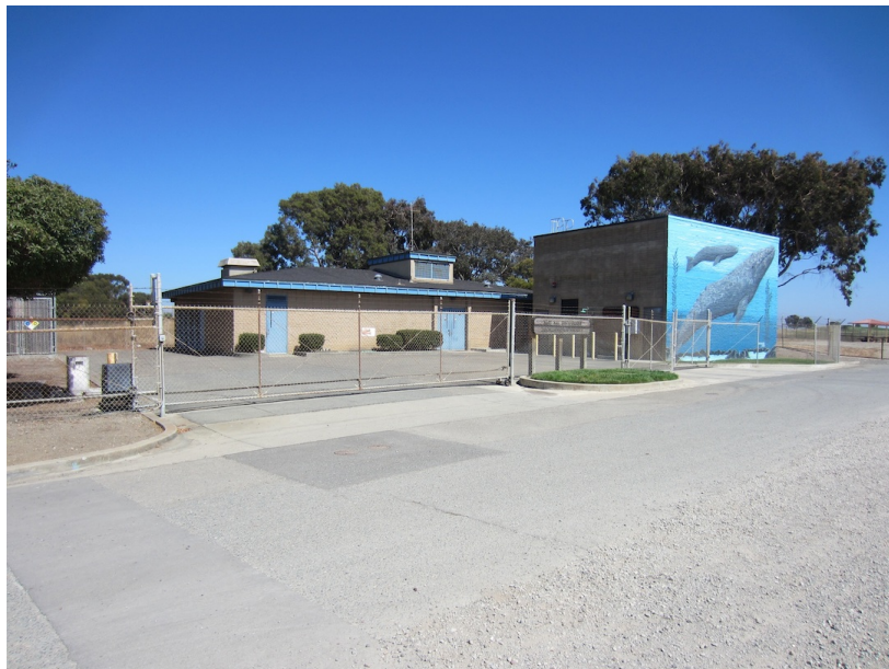
Figure 5. EBDA's Marina Dechlorination Facility.
