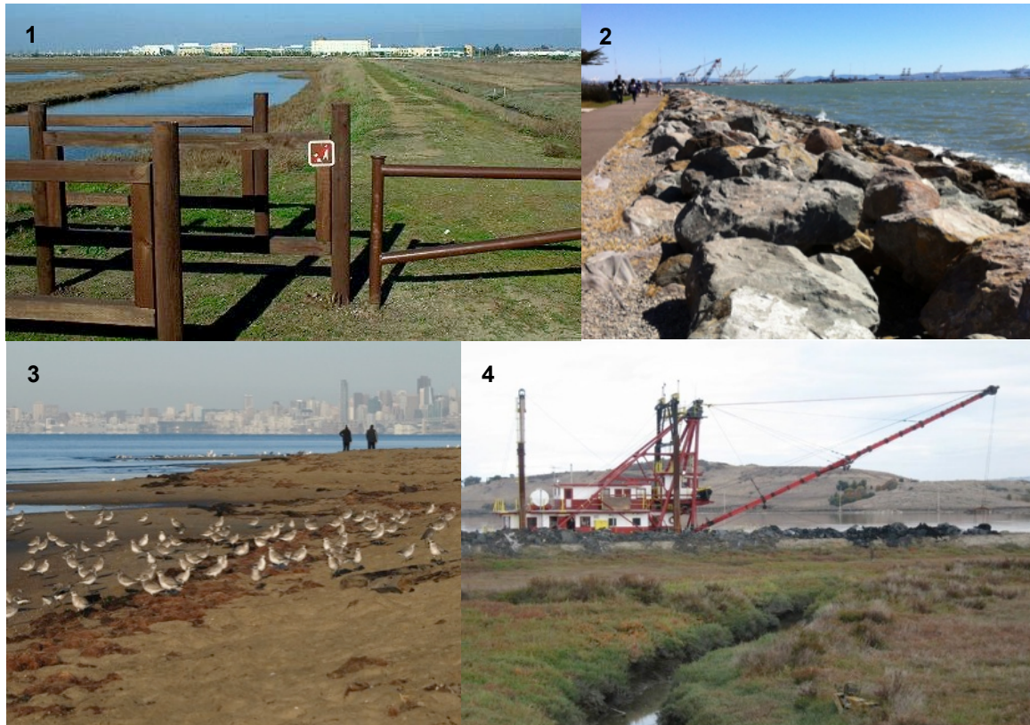
Figure 2. Shoreline categories in the ART project: 1) Engineered flood protection - levee with gate leading to LaRiviere Marsh (Source: Don Edwards San Francisco Bay National Wildlife Refuge); 2) Engineered shoreline protection - revetment along Emeryville's Marina Park; 3) Non-structural, natural non-wetland shoreline - Crown Beach (Source: Flickr Commons, Ingrid Taylor); and 4) Non-engineered berm in Eden Landing by Mallard, Hayward (Source: AECOM).
