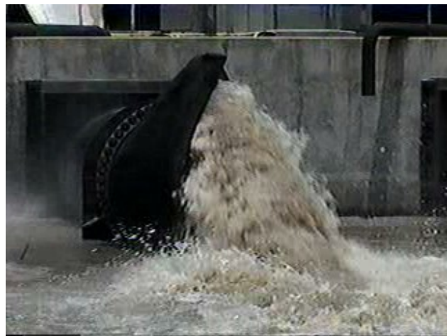
Figure 5. Duckbill check valve discharging water. Photo credit: Tideflex Technologies.
