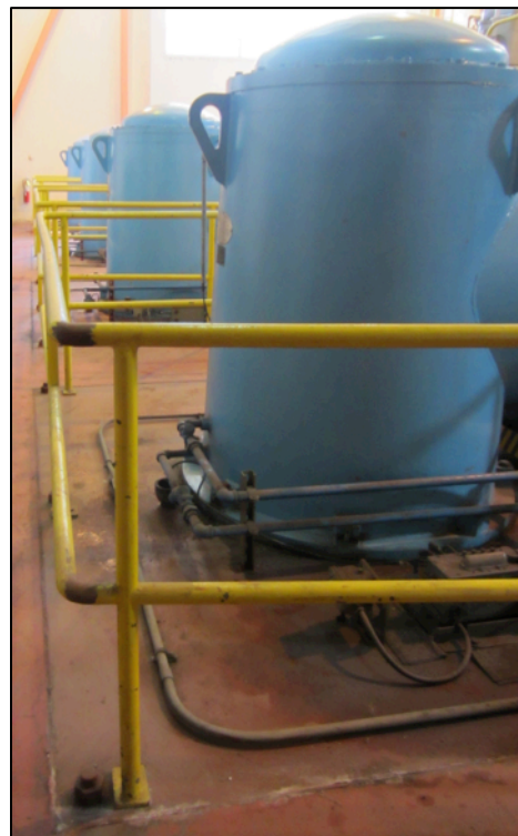
Figure 4. Pump components of the Ettie Street Pump Station, Oakland.
