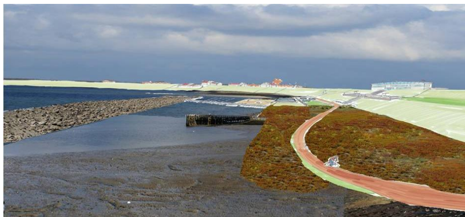
Figure 7.3 Rendering Of Levee Placed Out Into The Bay And Wetland Development Inboard of The Levee
