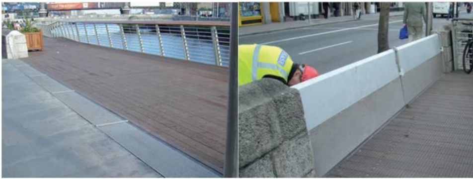
Figure 7.4 Demountable Floodwall Along Urban Waterfront
