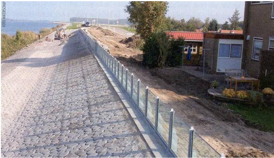
Figure 7.5 Glass Wave Overtopping Wall On A Levee
