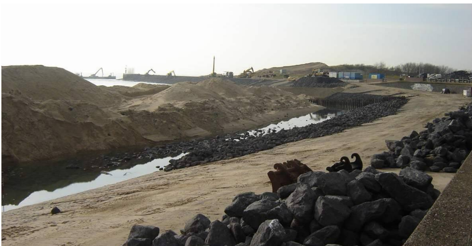
Figure 7.6 Raising Of Existing Levee
