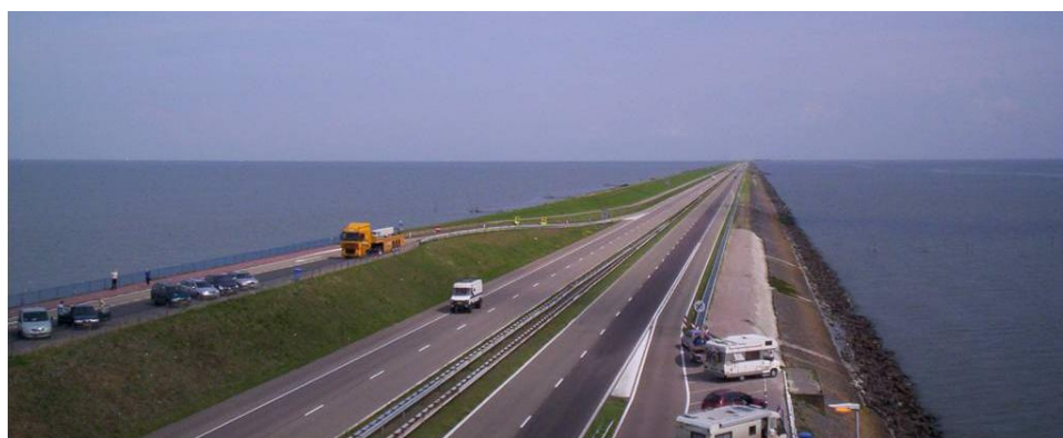
Figure 7.2 Freeway On Top Of A Levee
