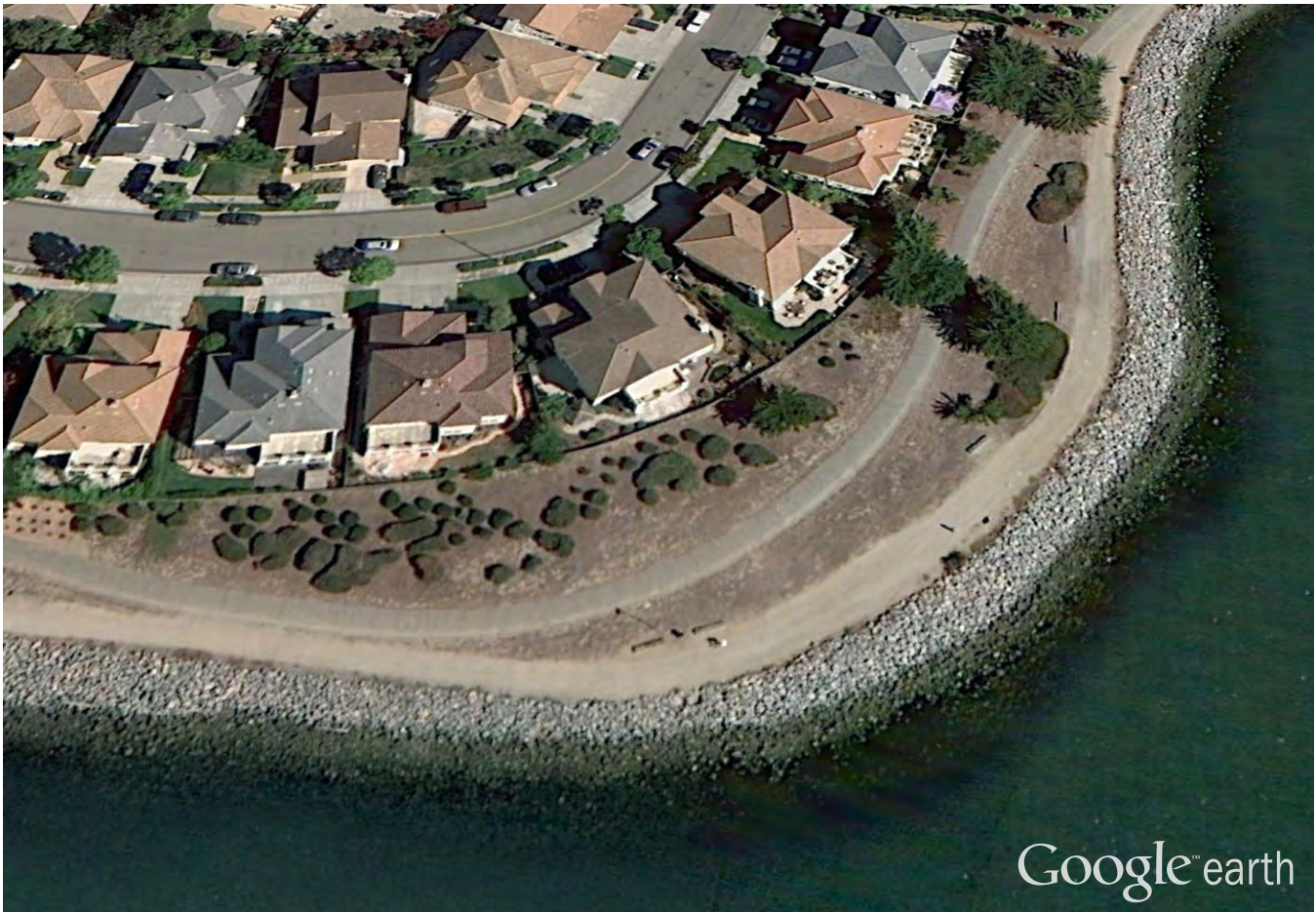
Revetment, Shoreline Park, Alameda
