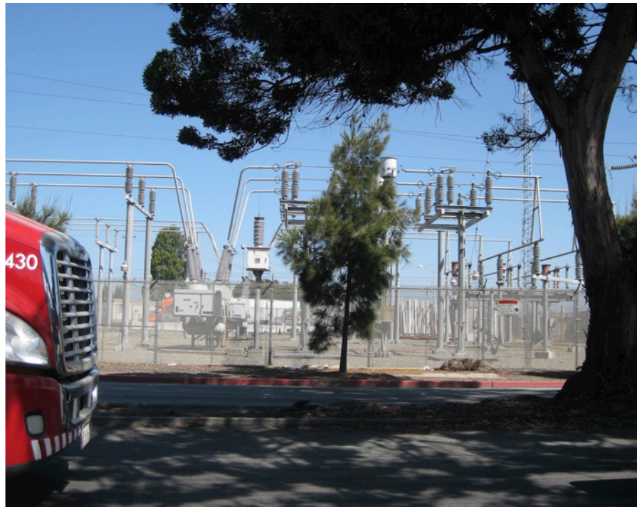
Figure 1. Energy assets evaluated include substations, which connect transmission and distribution systems and are a critical component of the electricity system.
