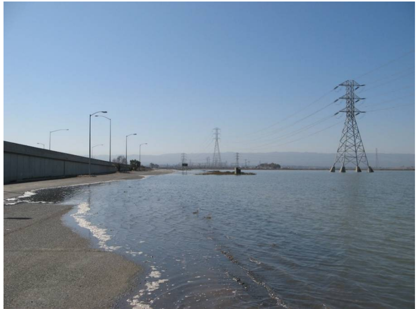
Electrical transmission lines on the Hayward side of the San Mateo-Hayward Bridge. Source: Rafael Montes, BCDC.
