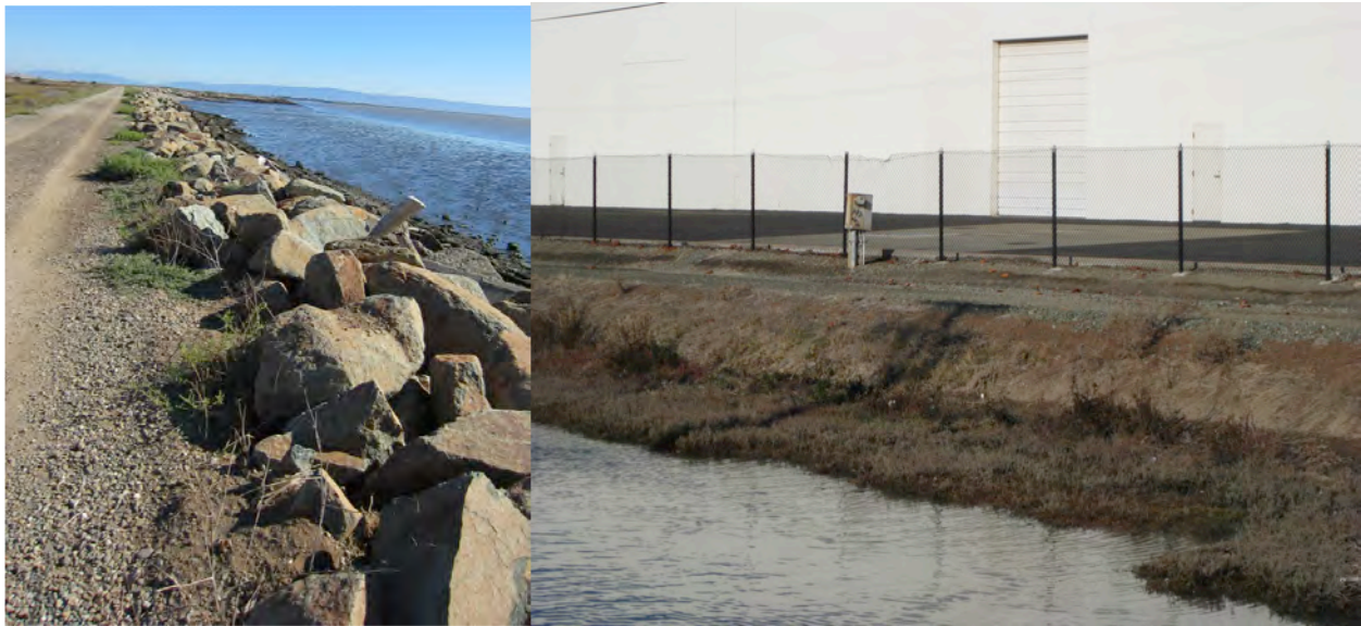
Photographs of representative segments of non-engineered outboard (left) and engineered inboard (right) levees within the study area.
