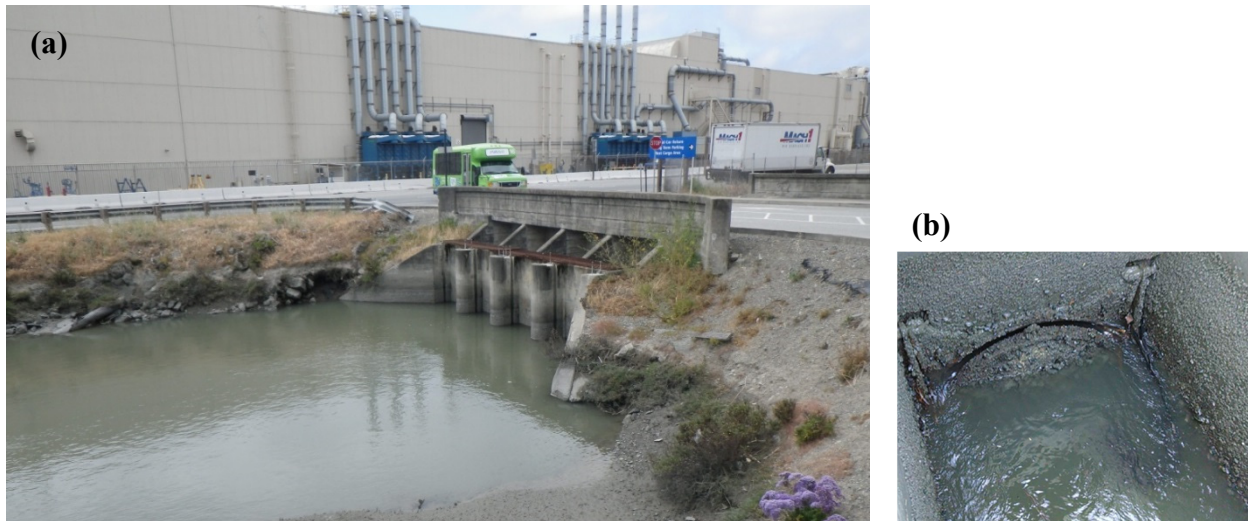
Figure 2-10. San Bruno Channel. (a) Tide gate Structure, Downstream Side (b) Flap Gate
