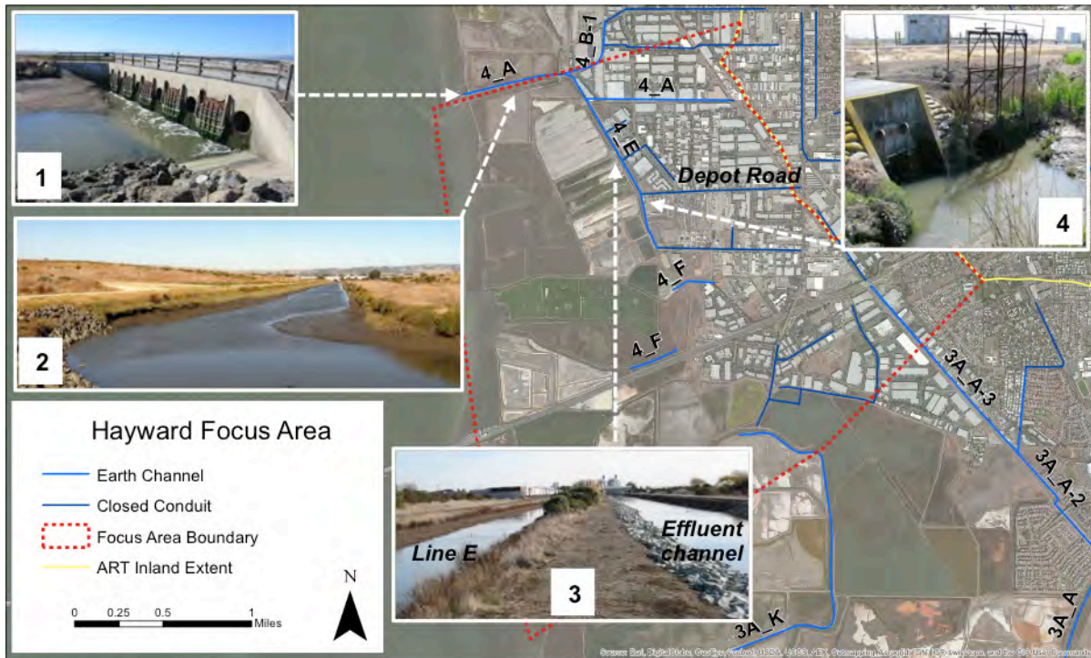
Map and photographs of the flood control system (all looking upstream): 1) Outfall structure at the Bay; 2) Line A channel extending from the Bay to the confluence with Line E; 3) Line E channel adjacent to commercial and industrial area and the Hayward Water Pollution Control Facility effluent channel (on the bayward side); and 4) water control structures at Depot Road.
