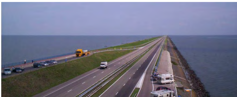
Figure 7.2 Freeway On Top Of A Levee
