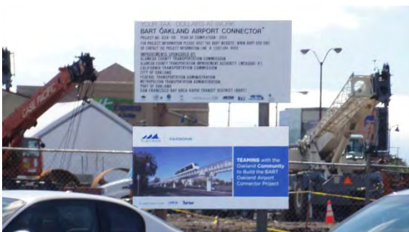
Future Oakland Airport BART Connector
