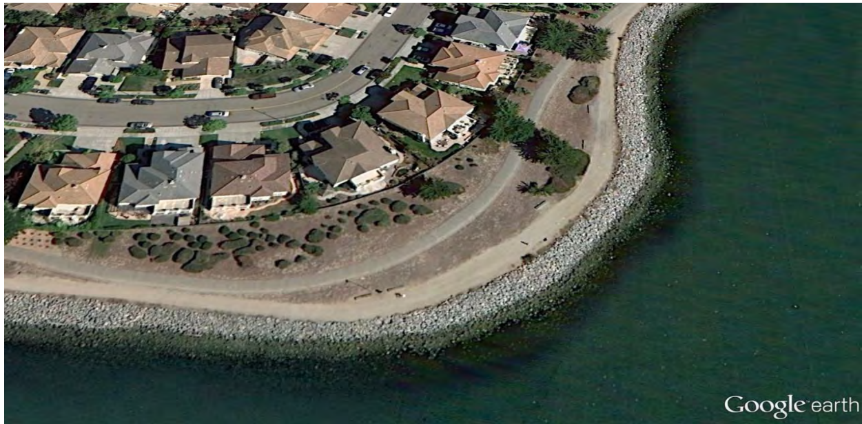
Figure 2.8 Revetment, Shoreline Park, Alameda
