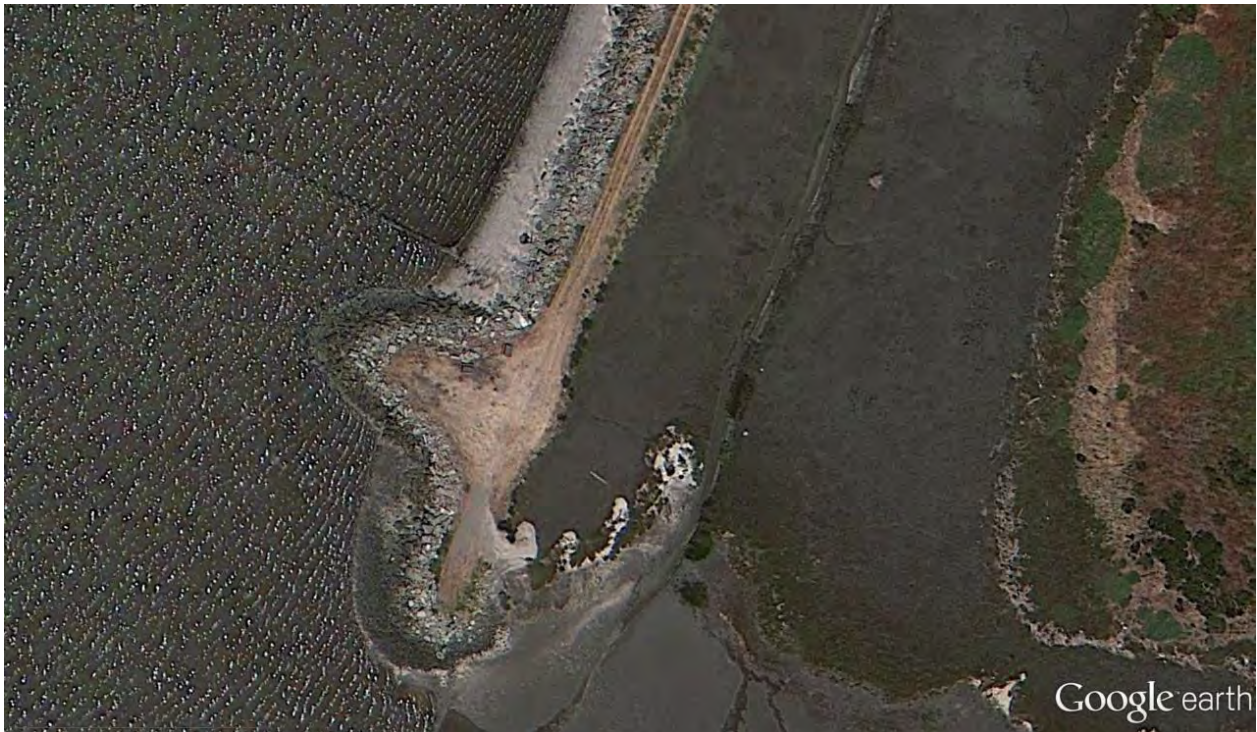
Figure 2.14 Nonengineered Berm with Riprap-Protecting Tidal Marsh from Wave Erosion, Hayward (see Hayward Marsh Figure 2.17 below under “Wetlands”)
