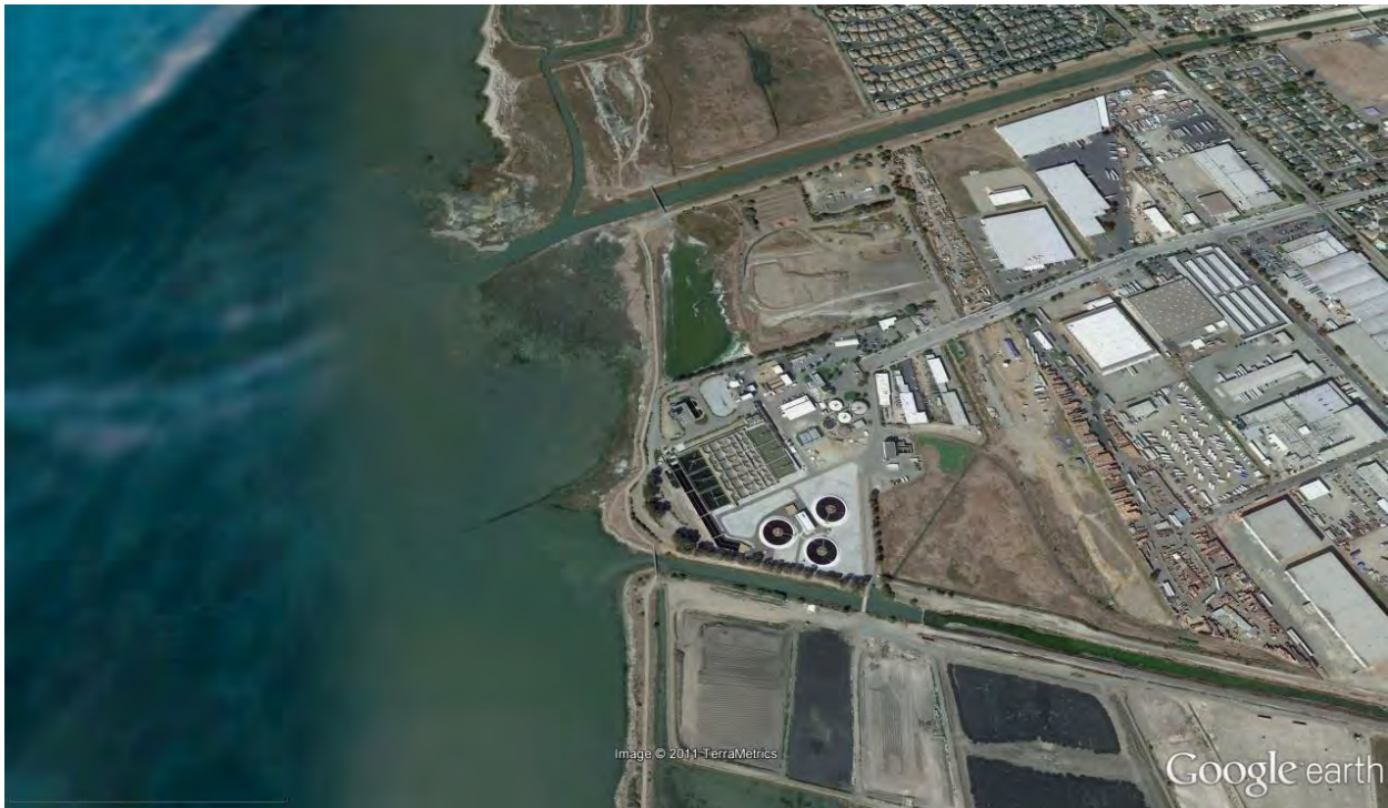
Figure 2.16 San Lorenzo Creek Tidal Flats, San Leandro (Some Inland Areas Have Riprap-Armored Shoreline; see Figure 2.21)
