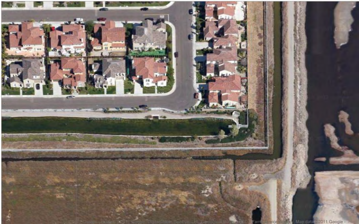
Figure 2.6 Flood Wall: Eden Shores, Landward of Eden Landing Complex, Hayward (Nonengineered Berm also Pictured to the Right of the Floodwall with Roadway as Berm Crest)
