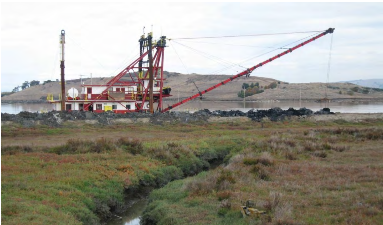
Figure 2.12 Maintenance of a Nonengineered Berm in Eden Landing by the Mallard, Hayward
