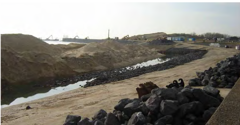
Figure 7.6 Raising Of Existing Levee
