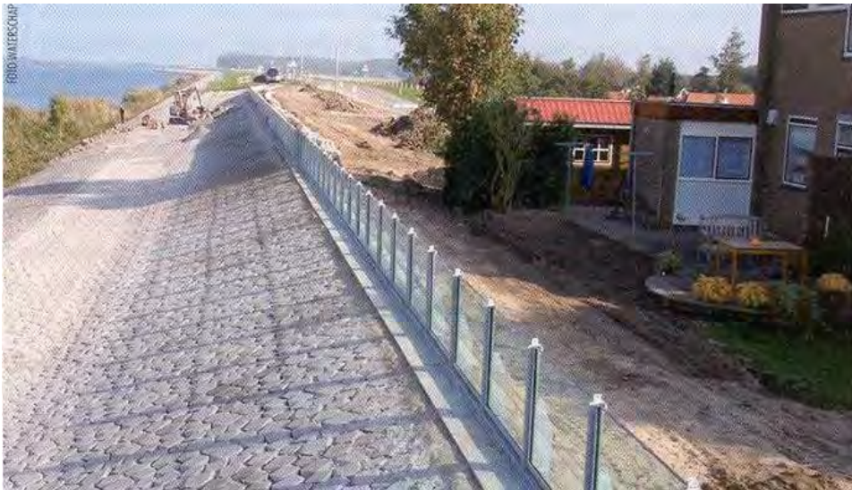
Figure 7.5 Glass Wave Overtopping Wall On A Levee
