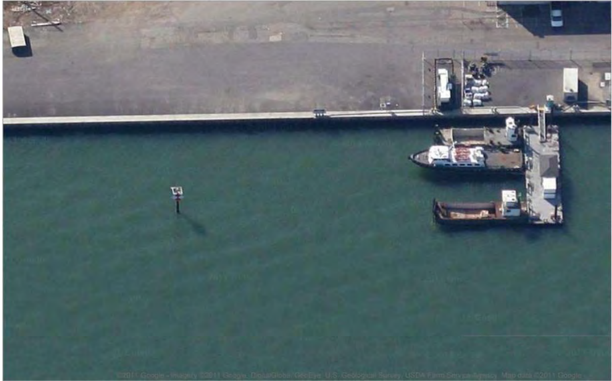
Figure 2.7 Bulkhead, Port of Oakland, Oakland
