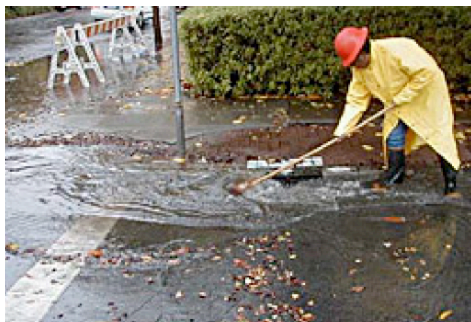
During heavy rains runoff can quickly overwhelm aging, undersized, or poorly maintained stormwater infrastructure. Source: US EPA.
