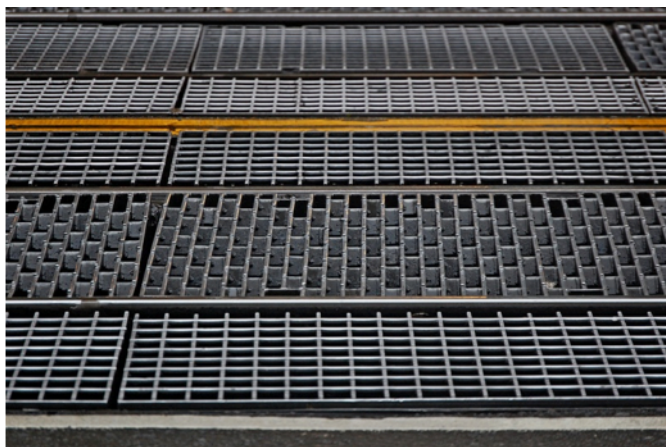
Figure 4. Example of BART street-level subway vents along Market Street, San Francisco (Source: http://nikdaum.com/news/10sf540big.jpg )
