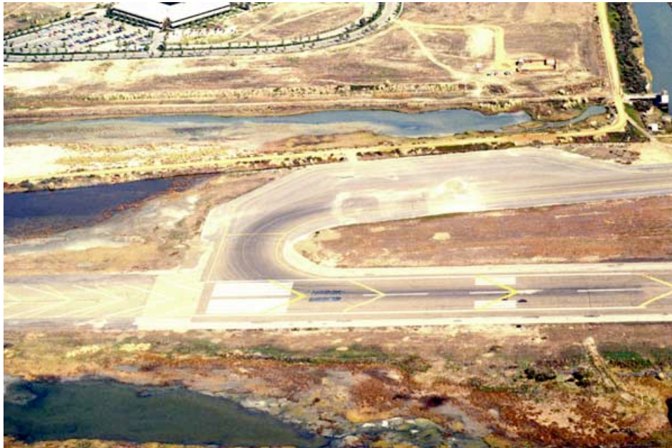
Figure 3. OAK's Main Runway after Loma Prieta Earthquake, with sand boils and cracks (above) and a close up of a sand boil on the main runway (below)
